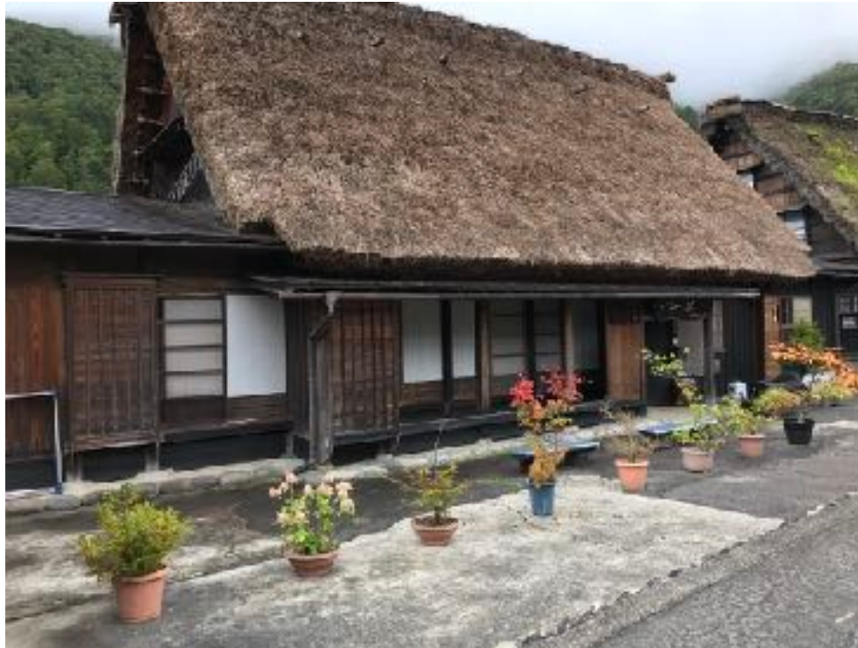
The scenic Shirakawa-go village (a UNESCO World Heritage site) is in the mountains of Japan. They get lots of snow, & their steep thatched roofs help shed the snow. Judy Maas
